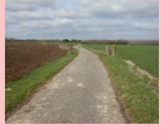
Tarmacked farm road with public right of way MIKE FAHERTY
